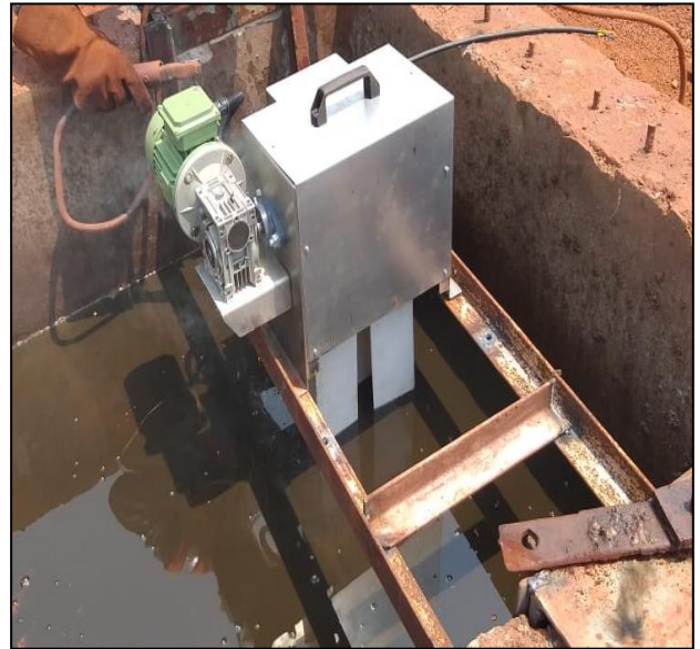
Photo# 17 : Effluent Treatment at workshop with Oil & grease trap pit and Oil skimmer
