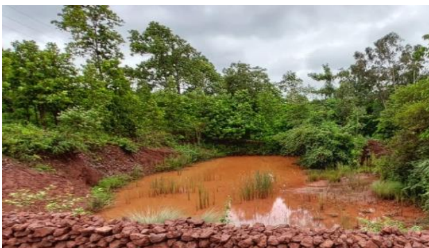
Photo# 7,8 & 9: Settling Pond, Check dam and check weirs for
