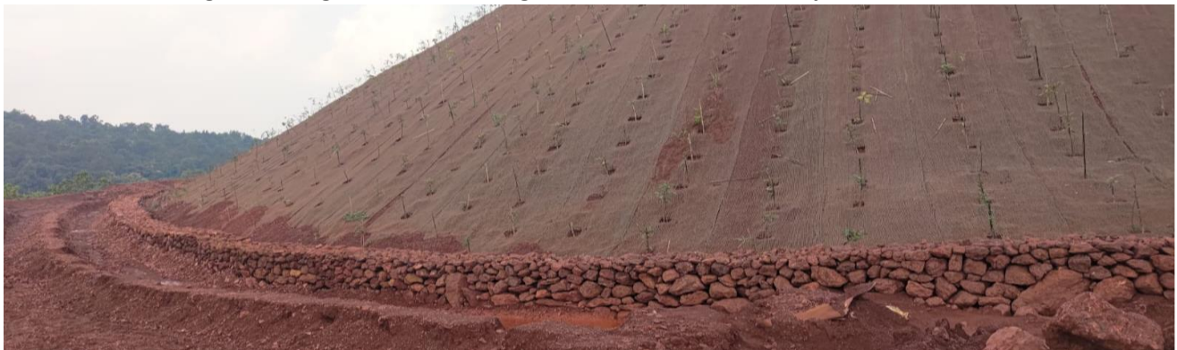
Photo# 15 Retaining wall and garland drain along the toe of Stabilised Dumps
